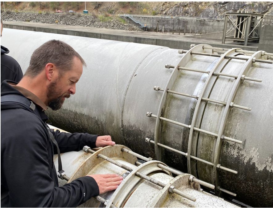
ENGINEER INSPECTING THE EXPANSION COUPLERS
