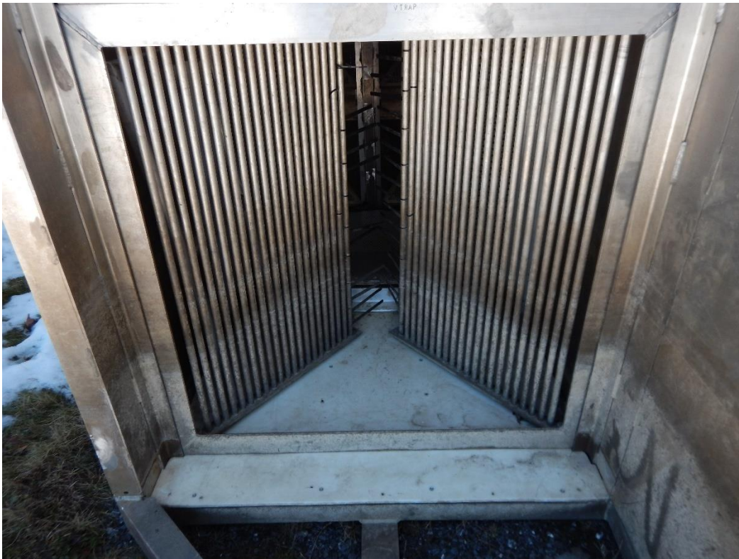
Figure 2. Entrance to the first stage of the trap (Vee-Trap section) of the Morpion Stream sea lamprey barrier.
