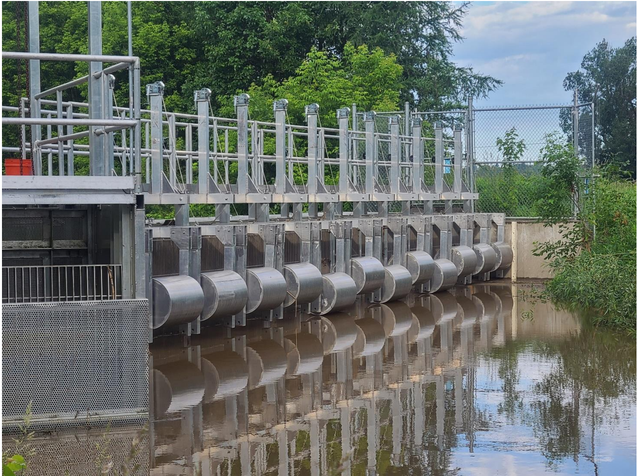
Figure 1. A picture of the barrel floats on the Morpion Stream sea lamprey barrier. This picture is looking downstream towards the barrier. This is considered high water (approximately 2 meters deep) When the water levels reach approximately 2.3 meters deep the lower barrels (3) will trip allowing those grates to drop downstream allowing the water level to drop. If the water level continues to rise additional barrels (9) will trip.
