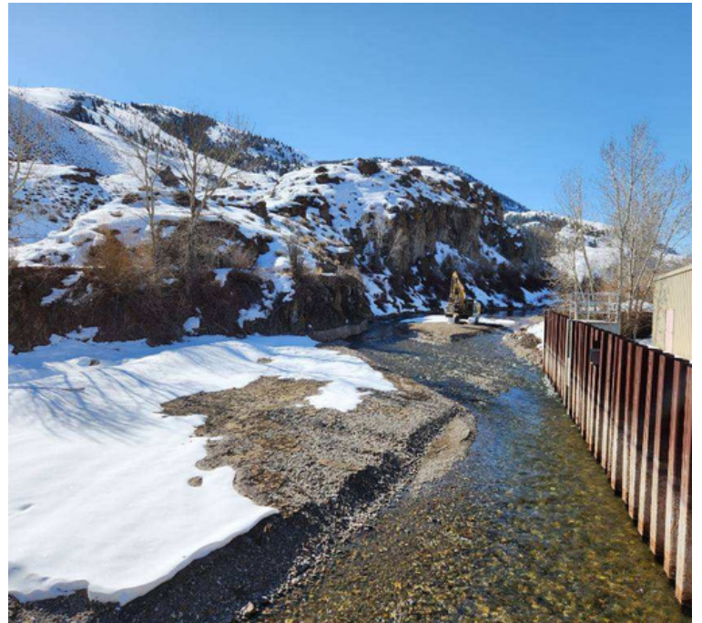
DEBRIS REMOVAL AT THE EAST FORK SALMON RIVER TRAP
