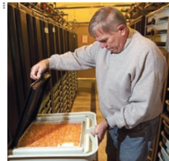
Tom Johnson from construction and design firm HDR checks the incubation stacks during the hatchery's commissioning.
