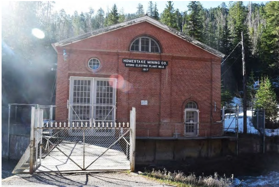
Figure 3. North face of LA00002055. View is to the south-southeast.
