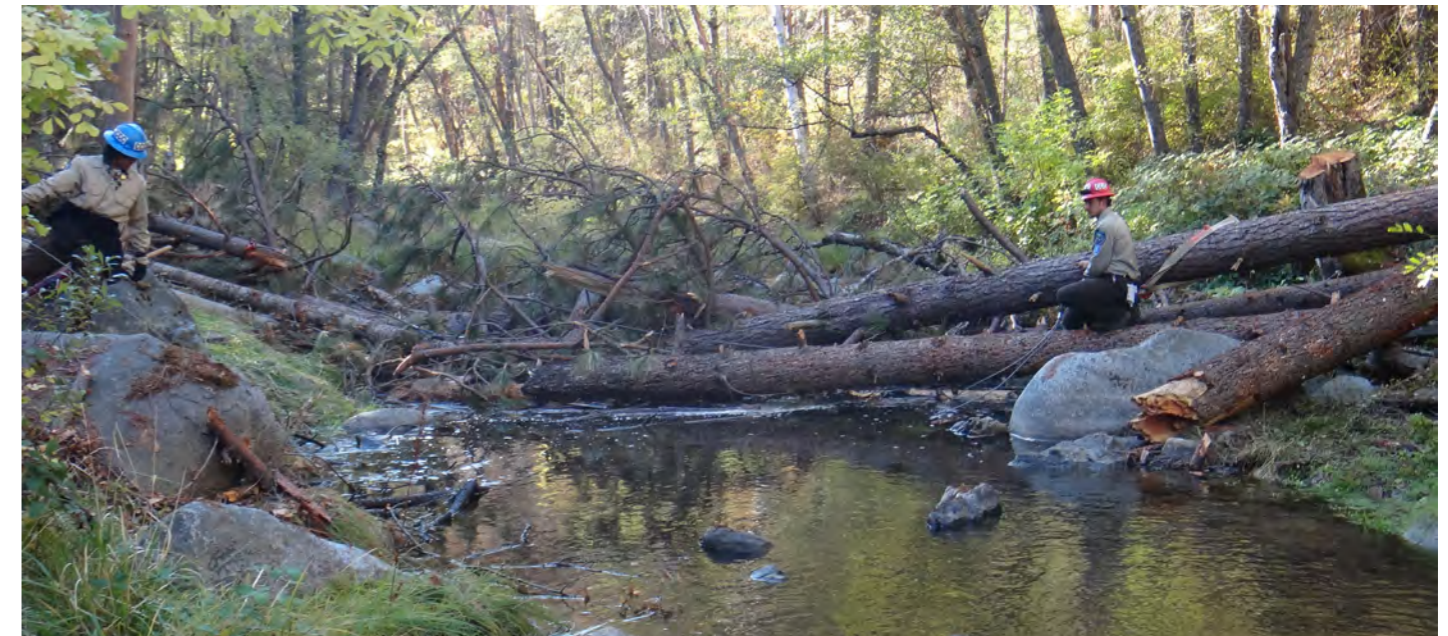
California Conservation Corps constructing Log Jam 2 on the Cottonwood Creek Accelerated Wood Recruitment Project Phase II. ©USFWS.
