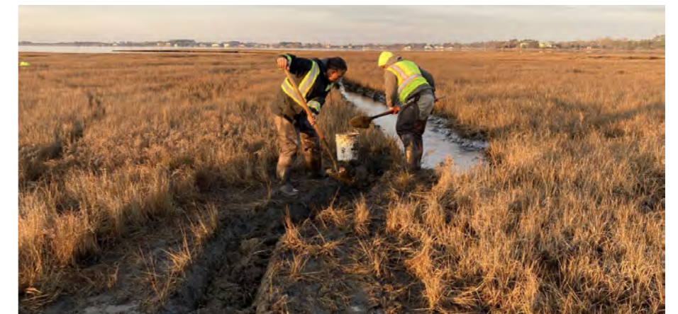
Contractors hand-digging a runnel at Rum Pointe. Photo by Katherine Stahl, USFWS.
