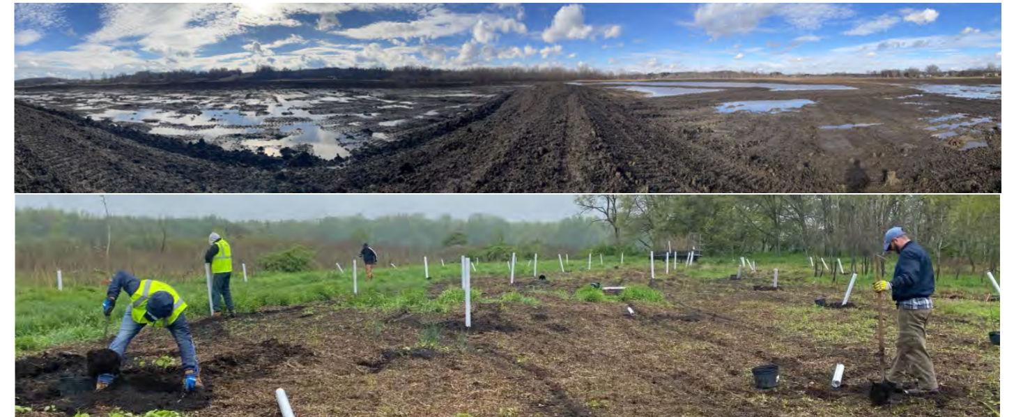
Restoration underway at the Western Reserve Land Conservancy. ©USFWS.
