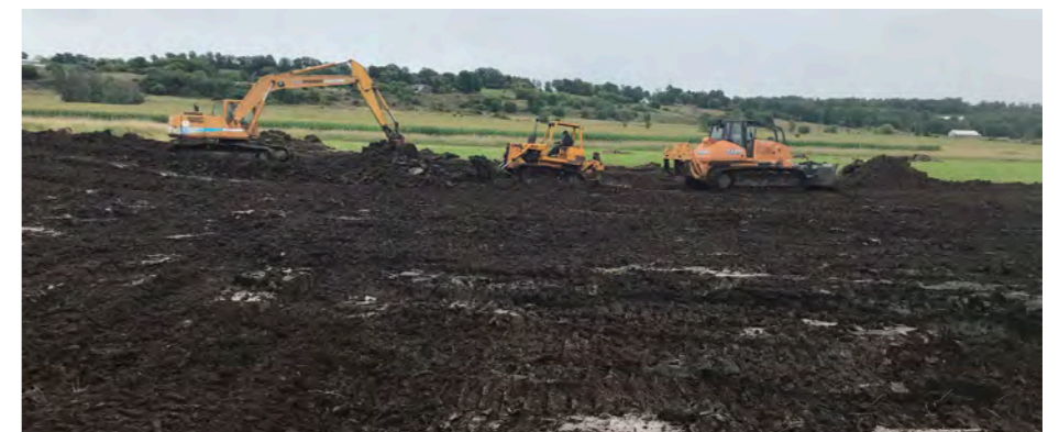
Heavy equipment excavating a depressional wetland. ©USFWS.
