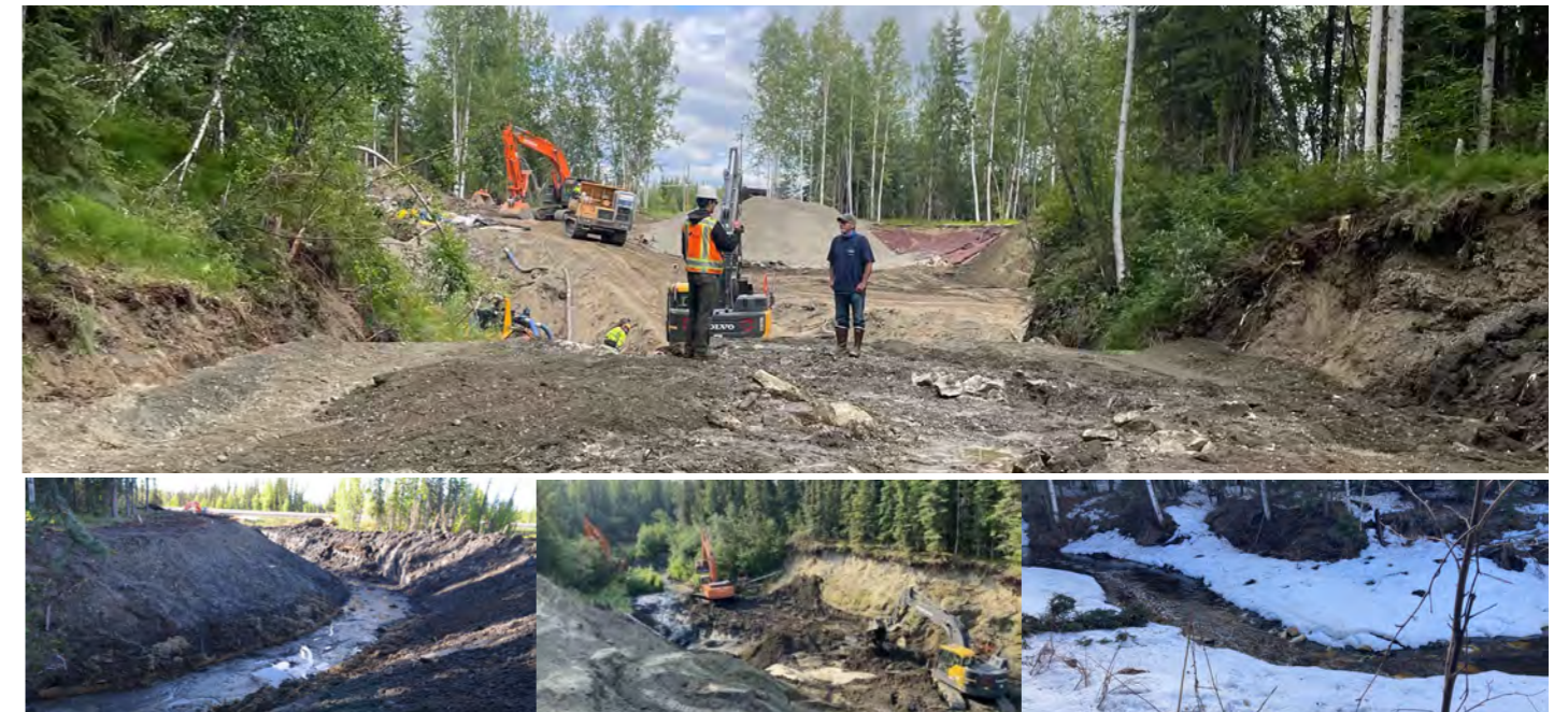
Happy Creek channel construction (top), active construction of stream channel (bottom left), site construction prep (bottom middle), Happy Creek fishway now connects to Cripple Creek natural channel (bottom right). ©USFWS.
