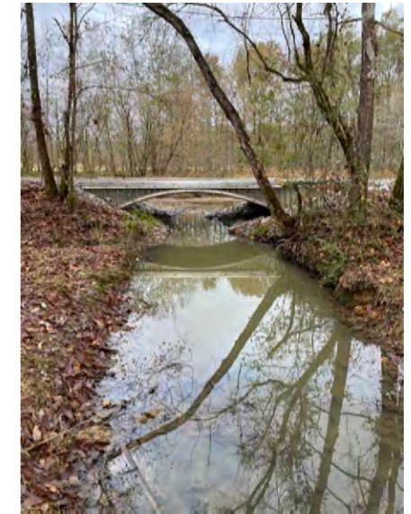
Left: Before restoration, Right: After restoration. ©USFWS.
