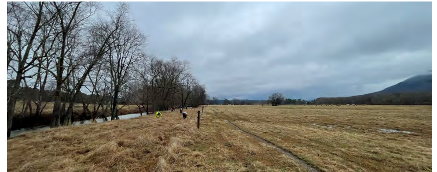
One of three designated low water crossings fortified during the project to permit cattle accessing water during the summer and accommodate rotational grazing practices on pastures occurring on both sides of Holly Creek. Photo taken by Joseph Kirsch/USFWS
