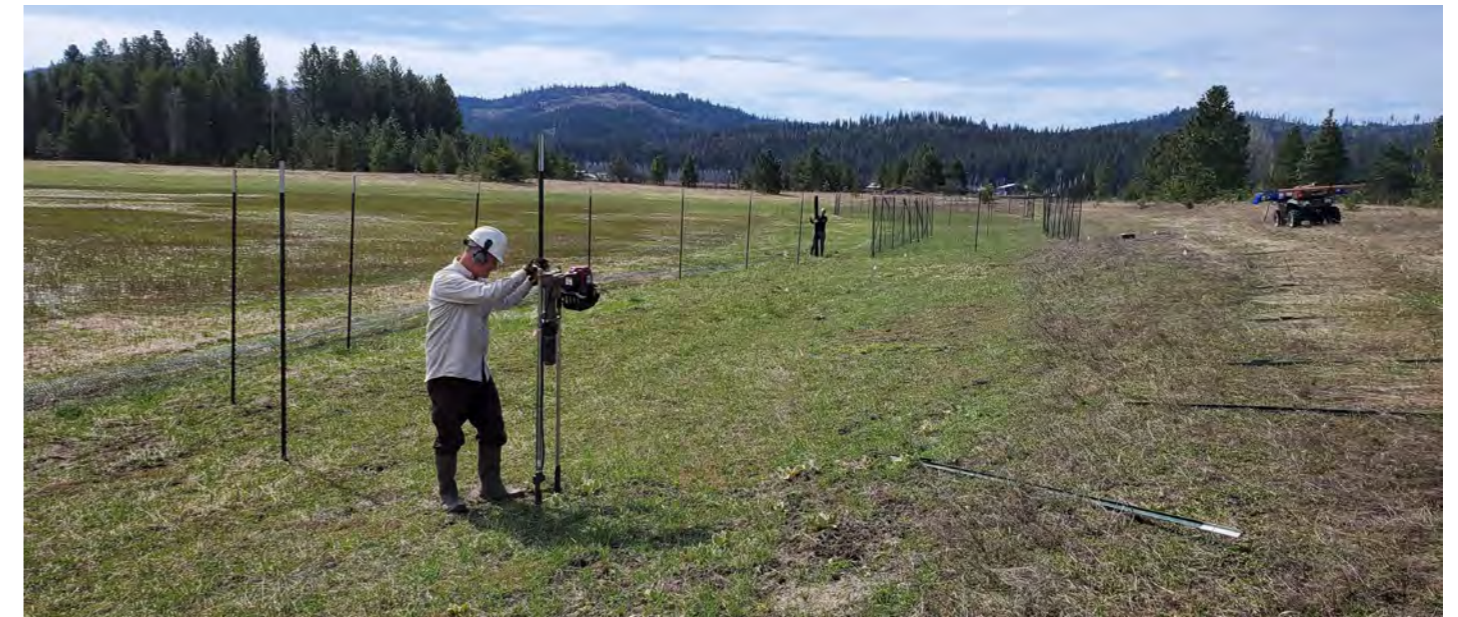
Installing 10 foot t-posts and 7 foot tall deer fencing to keep deer, elk, and moose from uprooting newly planted trees and shrubs. Photo credit: Ducks Unlimited.
