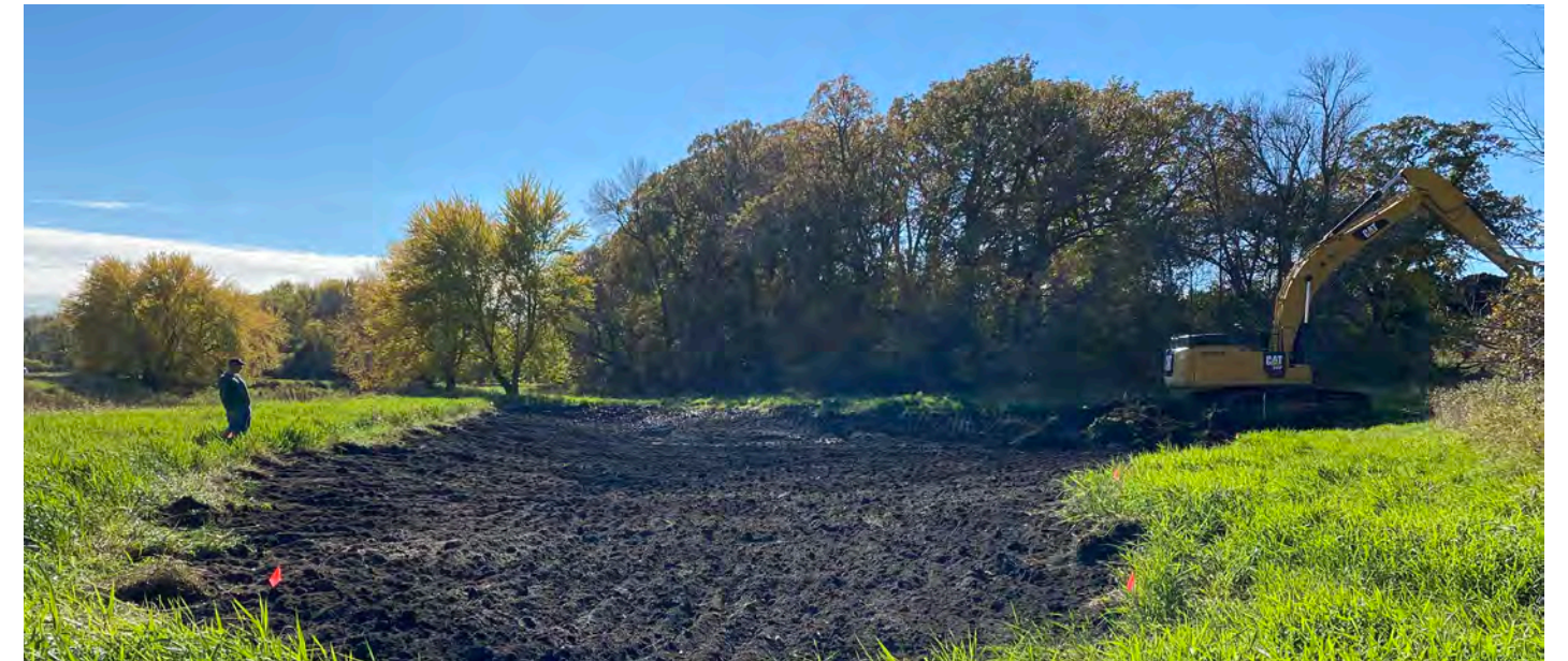
Restoration in progress. ©USFWS
