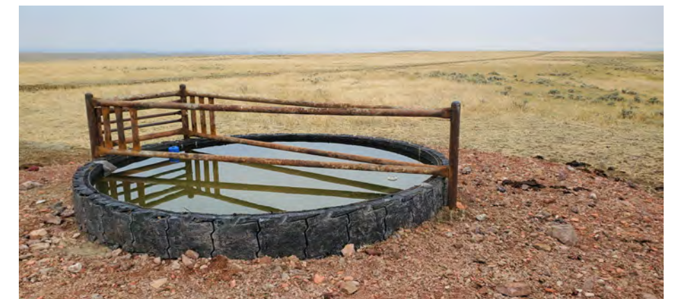
Completed tank with wildlife ramps installed installed. ©USFWS
