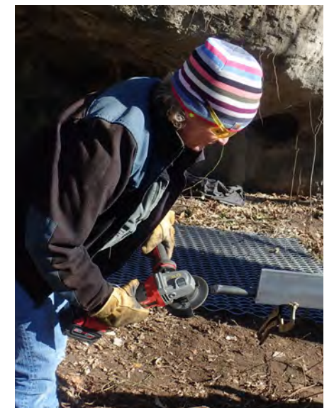
Toby Gate crew during construction at project site. ©USFWS
