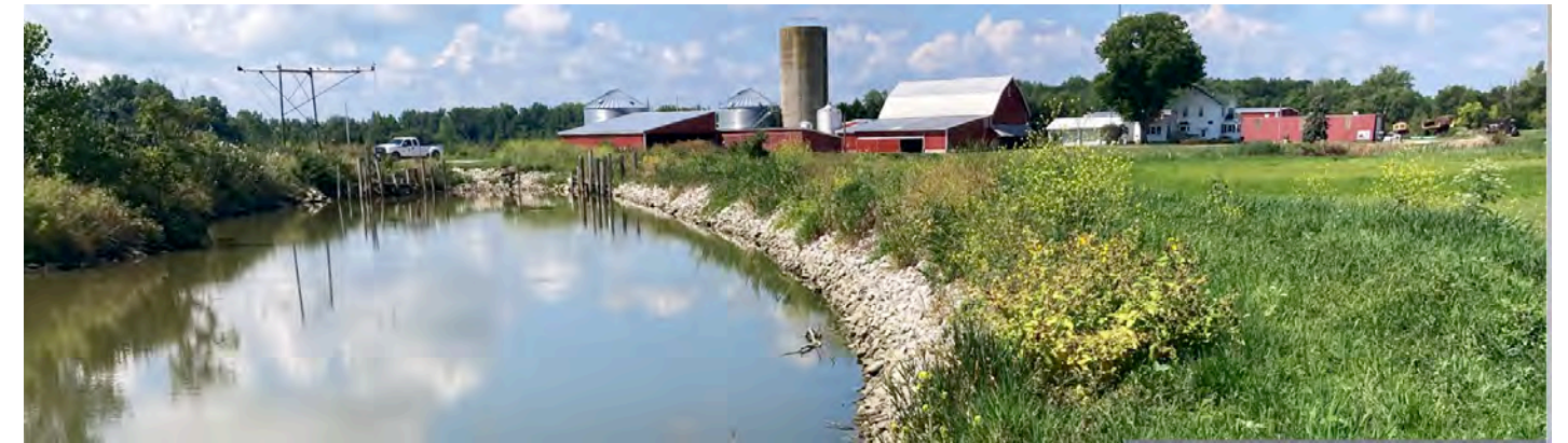
"After" restoration / completed project area where water now reconnects from Muddy Creek into the watershed. ©USFWS
