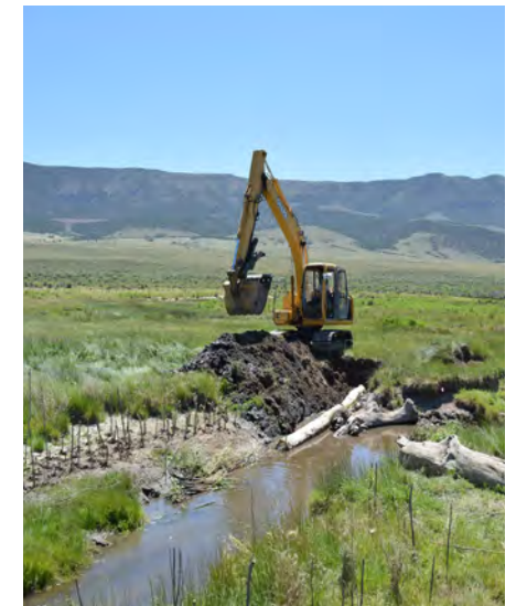
Heavy equipment used for instream restoration. ©USFWS.
