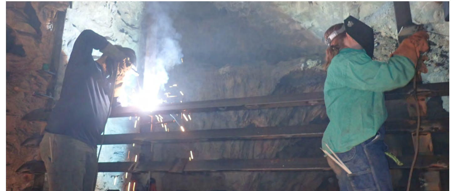
Volunteers welding at Toby Cave Gate project. ©USFWS
