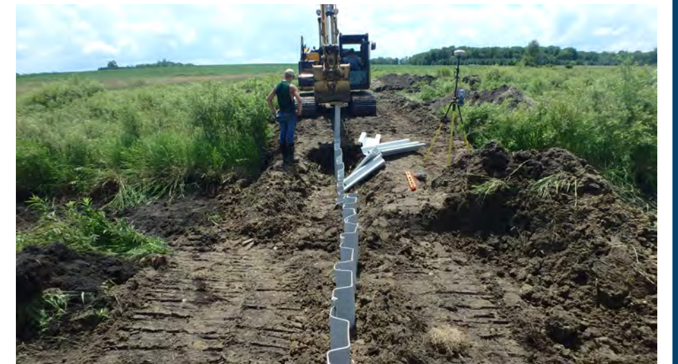
During restoration at project site. ©USFWS
