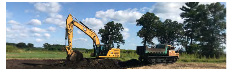
Aerial view of project site (above). Restoration in action (below). ©USFWS
