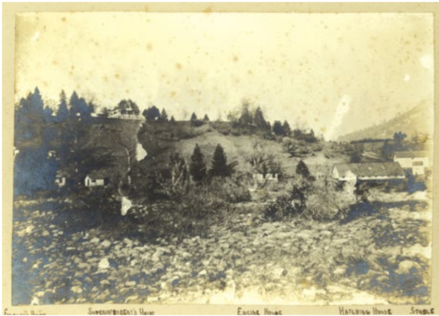
The U.S. Fish Commission built its first hatchery, the McCloud Hatchery, in 1872 in California. It set the stage for successful salmon rearing and planting for more than 400 other fisheries facilities during the next 150 years. The Service renamed the McCloud Hatchery as the Baird Hatchery after the first Commissioner, Spencer F. Baird. After the installation of a dam, the former hatchery site now lies under the waters of Lake Shasta. National Fish and Aquatic Conservation Archives/USFWS
