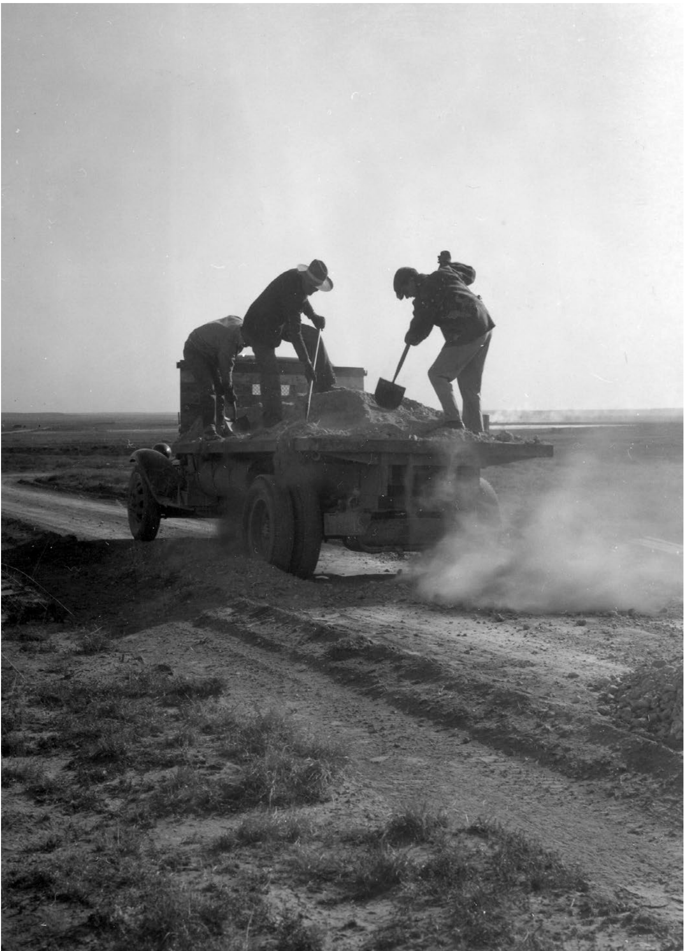
Works Progress Administration (WPA) workers lay road gravel at Dexter Fish Cultural Station ca. 1936 from a GMC truck. National Fish and Aquatic Conservation Archives/USFWS
