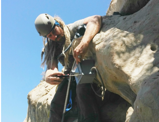
Photo 2.4.3: Supervisory Wildlife Biologist, Joseph Brandt, installs camera equipment outside the cavity at KR15. Photo Credit: Josh Felch, USFWS.
