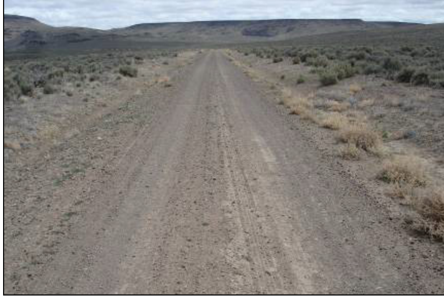
Photo 1.5 Disturbance from regular grading along road shoulders spreads and creates ideal growing conditions for many non-native invasive plants such as Russian thistle, Halogeton , and cheatgrass.
