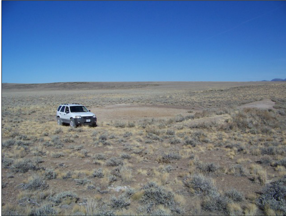
Figure 3. Typical stock pond; note the small earth dam at the right to impound water.
