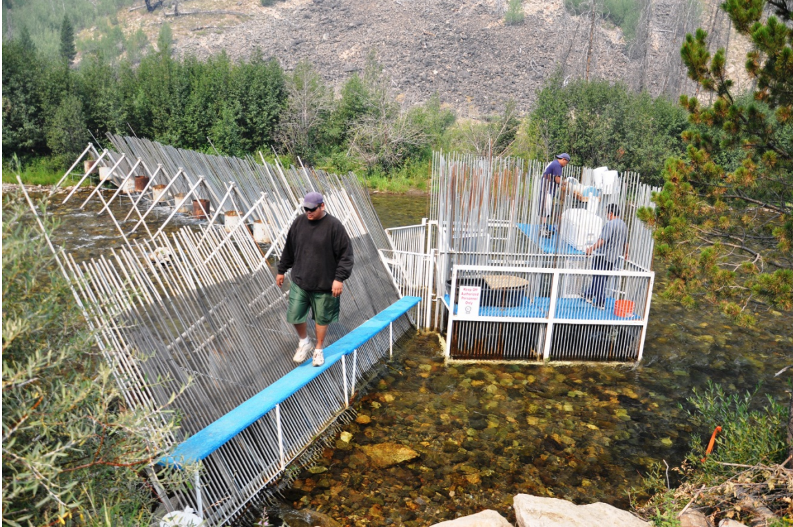
Figure 10. Pole Flat weir, catwalk, fish trap, live-wells, and work station.
