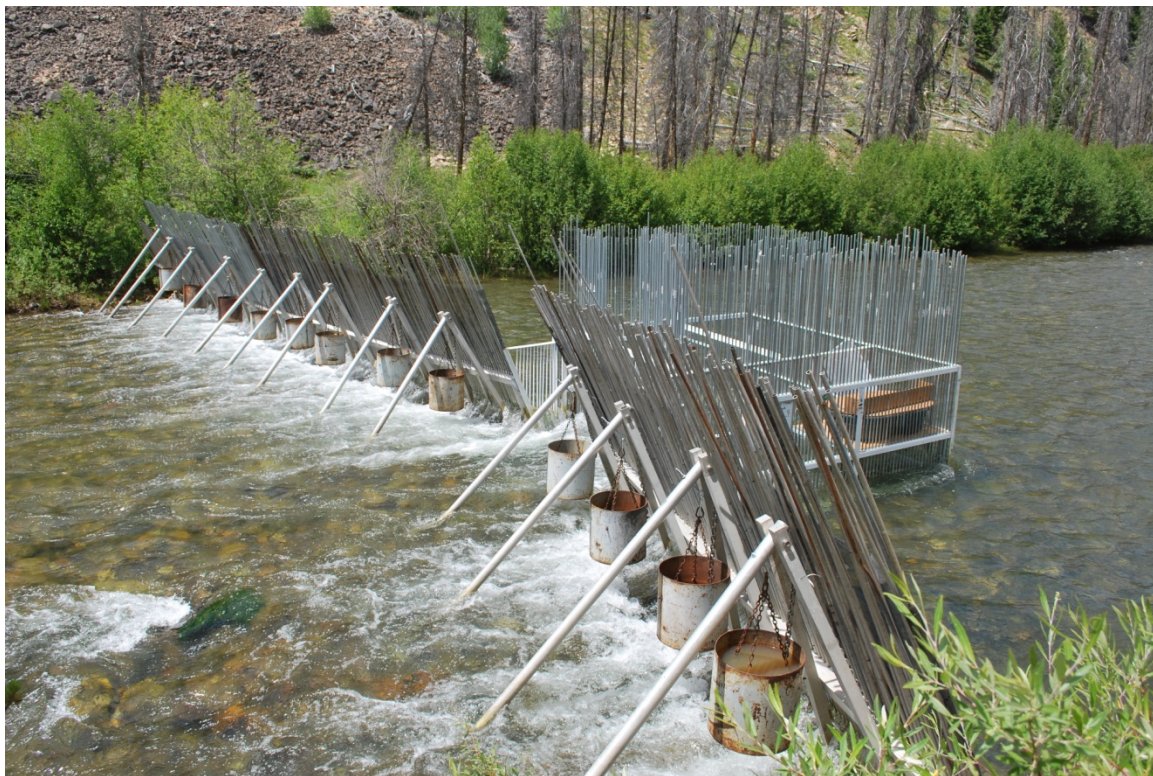
Figure 2. Pole Flat Weir.
