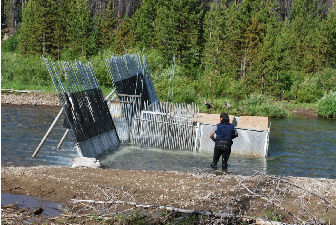
Figure 4. Five Mile Weir and Trap Box.
