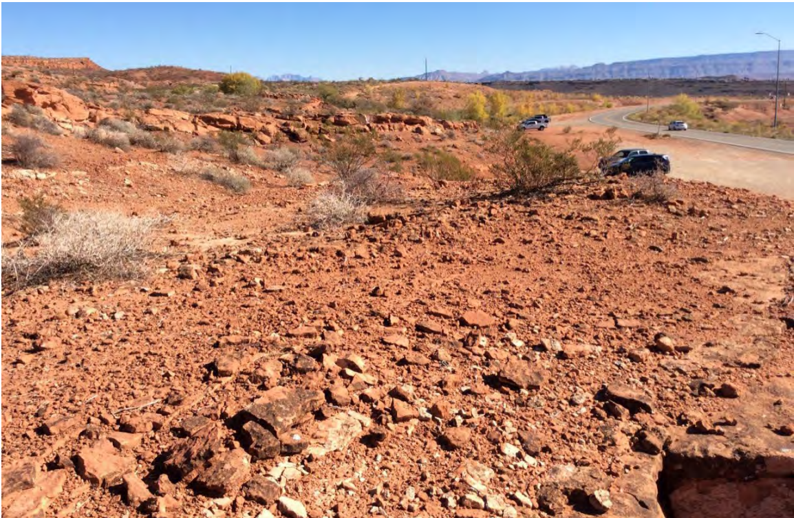
Photo 12. View east along Washington Parkway/Buena Vista Boulevard, showing unpaved roadside parking associated with the Grapevine Trailhead on the left side of the road.
