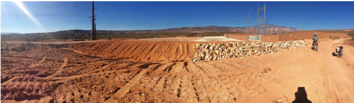
Photo 16. View of the electrical substation in the central portion of the Project area, looking west. This area is highly disturbed.
