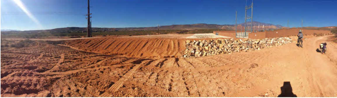
Photo 12. View of the electrical substation in the central portion of the Project area, looking west. This area is highly disturbed.
