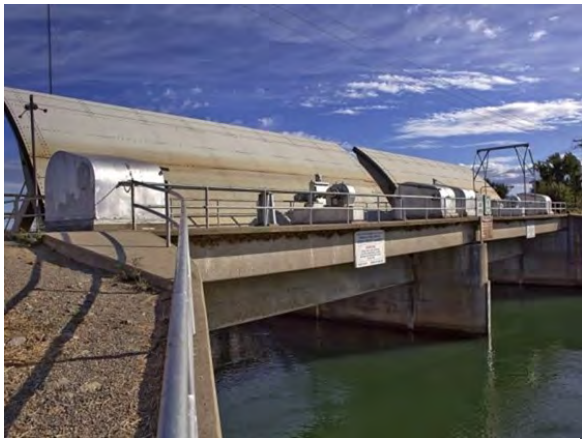
Fig. 3 - Closures of the Delta Cross Channel Gate prevents entrainment of many fish into the poor habitat of the central and south Delta and reduces salvage.
