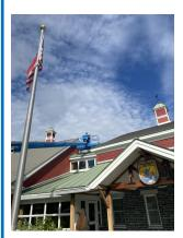
A four-person Great American Outdoor Act Deferred Maintenance Strike Team spent two weeks working on the exterior of the Nulhegan Basin Office/ Visitor Center. The maintenance crew rebuilt the cupolas, replaced most of the trim along the roof line/windows, replaced rotten clapboards and re-flashed areas that required attention. A big thank you to the New Hampshire crew for their support of the Conte Refuge.
