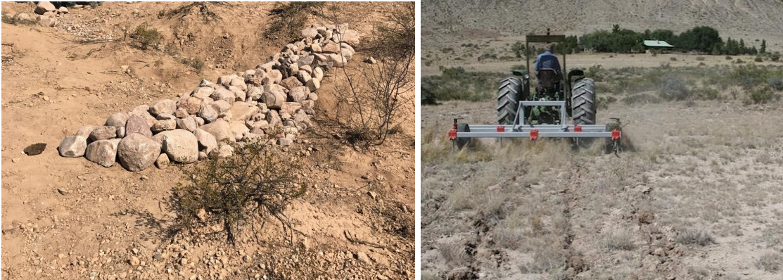
Rock erosion control structure (left) and keyline subsoil plowing (right), pictures courtesy of Watershed Management Group
