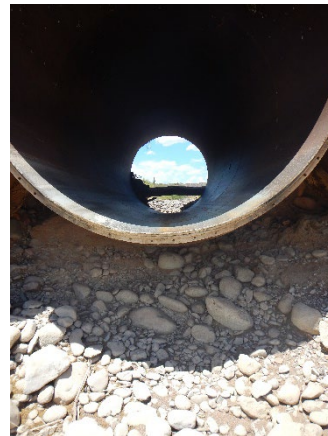
Photo 21. Eye level view of culvert at East del Chi Dr crossing, 7/28/20.
