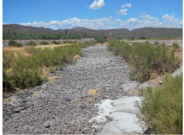
Photo 17. View upstream of channelized reach at East del Chi Dr crossing, 15.2 river miles upstream of A-Cross Rd, 7/28/20.
