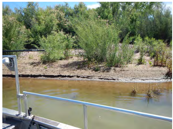
Photo 78. EF2 right bank (north).
