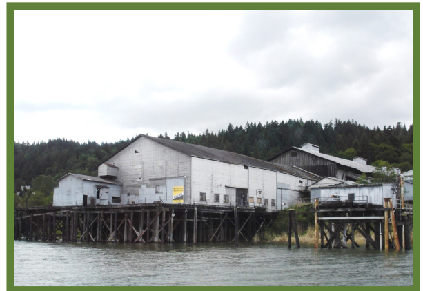
View of the Linnton Mill site from the Willamette River, prior to demolition of the buildings and docks.
