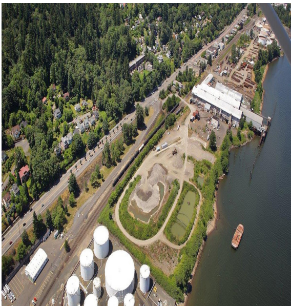
Aerial photo of the project site before restoration.
