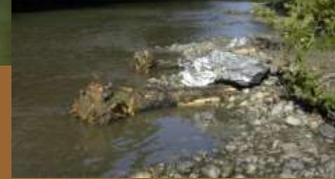
Habitat restoration techniques utilized a natural channel design and installation of rock vanes, log vanes, and large woody debris to provide a substrate for macro invertebrate production and cover for juvenile fish. This project will halt the excessive bank erosion, restore stable natural river dynamics and provide new fish habitat.
