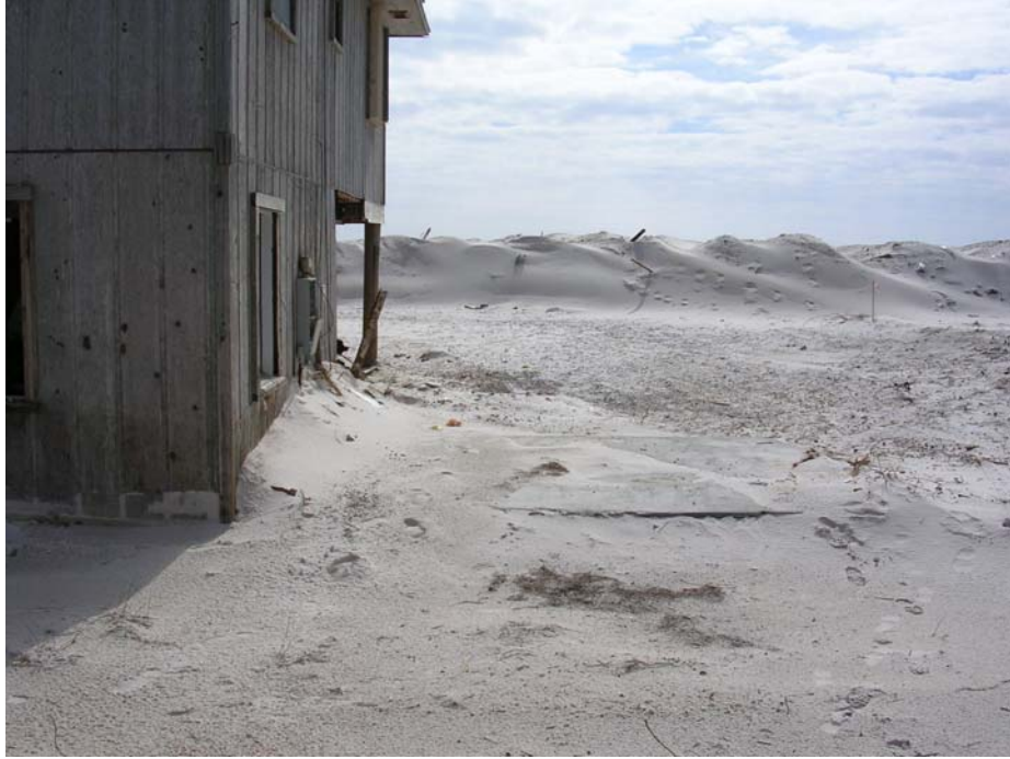
View south depicting west side of property
