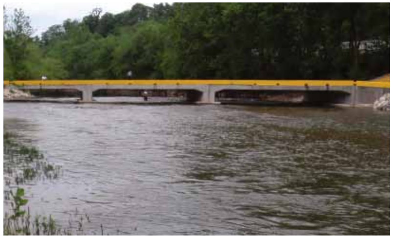
New Wiley Drive Bridge
