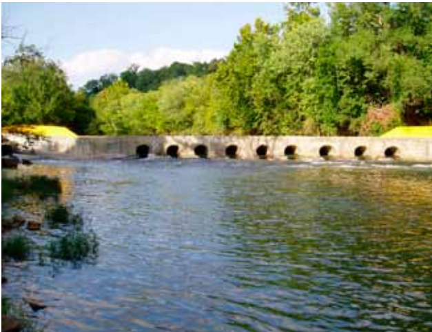
Wiley Drive Bridge Before Demolition
