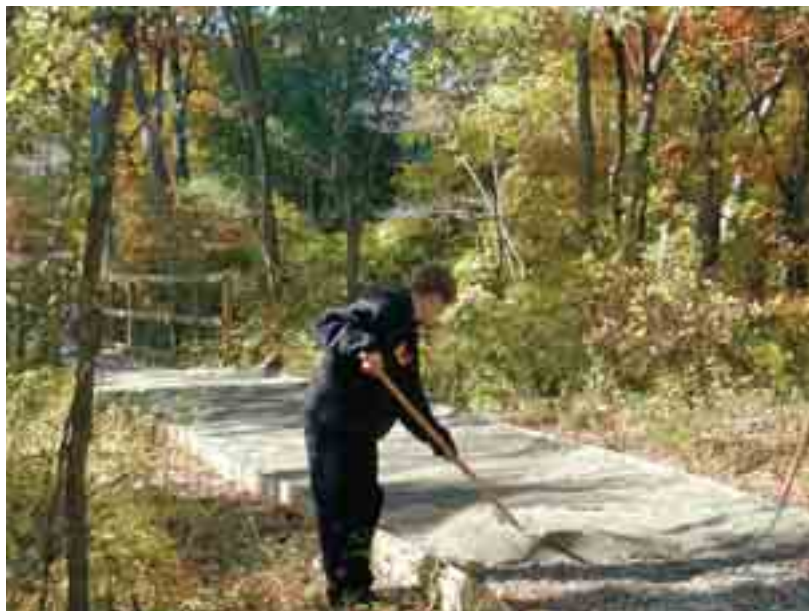
Volunteer helping to construct trail: USFWS
