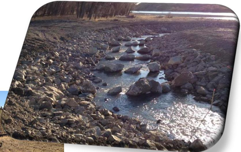
Figure 4. Restored lower reaches of bypass channel with improved slope. *YCCD photo.*
