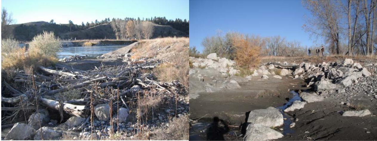
Figure 2. Debris jam at upper end of bypass channel (left), and siltation in lower end of channel (right).
