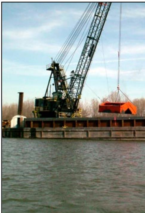
*A specially designed clamshell dredge bucket limited resuspension of sediment.*
