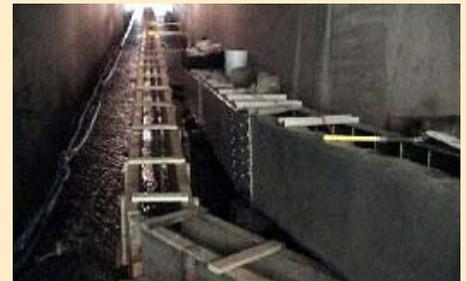
**Installation of this step-pool fishway structure at Grand Portage Creek in Minnesota reconnected 3.5 miles of spawning and nursery habitat for coaster brook trout.**
