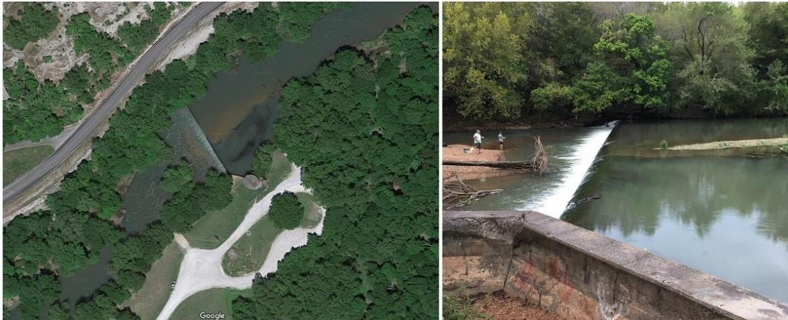
On the left is the overhead view of the Lime Kiln dam, the right picture is taken from the public use area on the left descending bank of Shoal Creek. Rock would be placed downstream of the dam.
