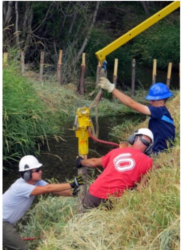
*Triple Creek team members and helper install a beaver dam analogue post using a pneumatic hammer.*
