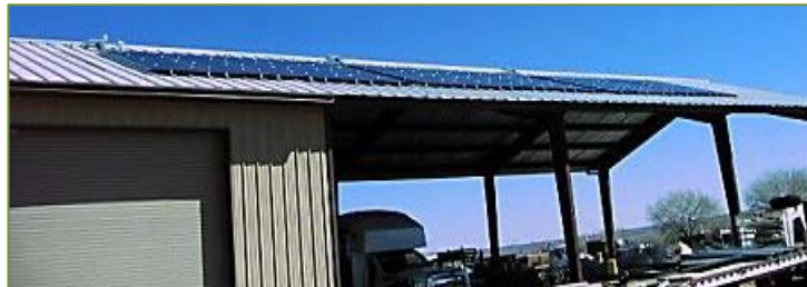
PV Array Vehicle Maintenance Shop – Bosque del Apache
