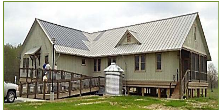
Photovoltaic System – Panther Swamp NWR
