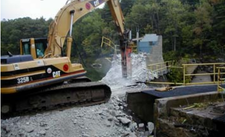
Smelt Hill Dam removal Presumpscot River
