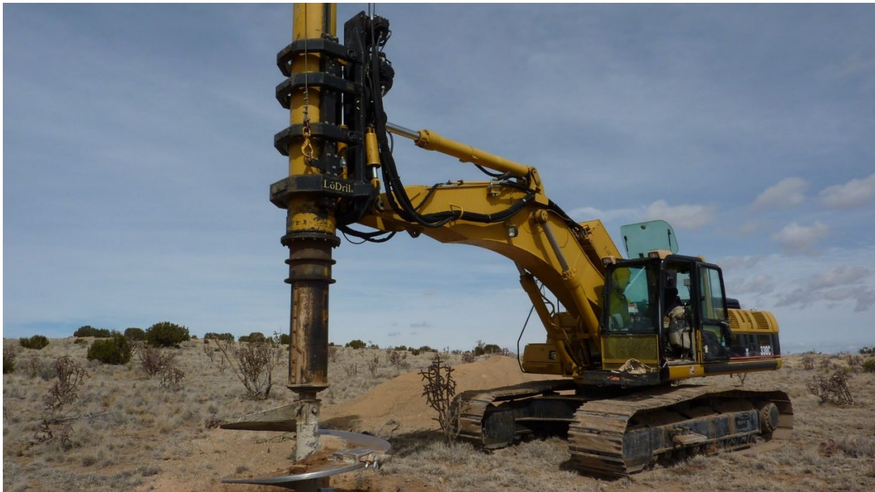
Figure 2 Pole Augering Example
