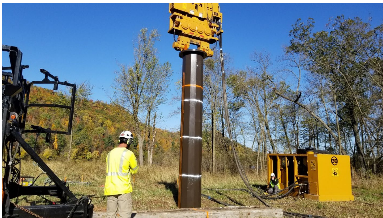
Figure 5 Example of pile driver and pile
