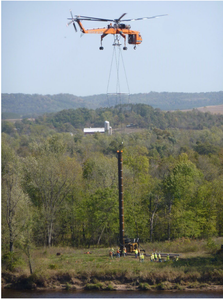
Figure 3 Helicopter positioning pipe pile above ground
