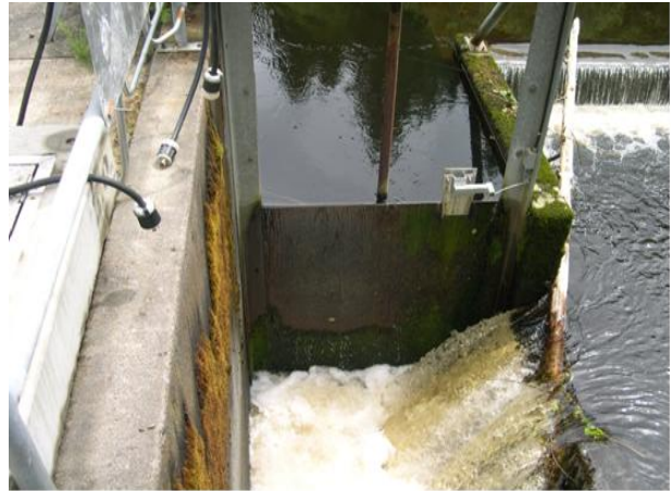
Photo 4. Cook Creek main intake diversion control gate.
