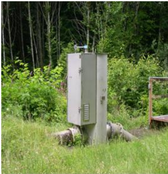
Photo 7. Siphon system priming structure.
