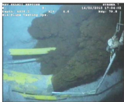
Figure A-4: Images showing the end of the riser pipe, left image showing riser pipe with oil flowing, right image shows end of riser with no oil flowing (FRTG 2010).
