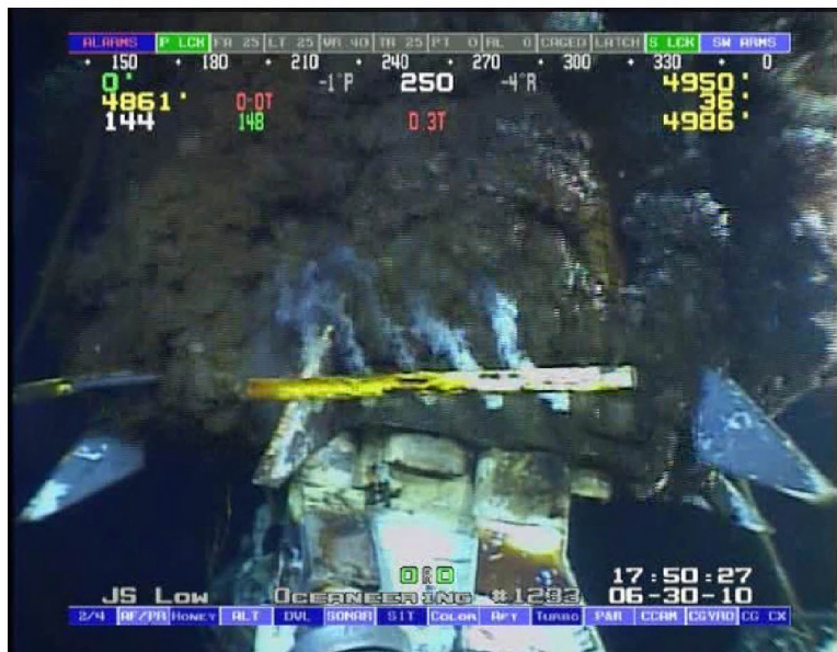
Figure F-3: ROV image of dispersants being applied by the trident (foreground) to oil escaping from the cut riser above the BOP and flowing around the top hat, June 30, 2010. The white plumes along the tine of the trident are the result of dispersants being sprayed through small holes on the inner face of the tine.
