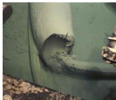
Figure A-4: Images showing the end of the riser pipe, left image showing riser pipe with oil flowing, right image shows end of riser with no oil flowing (FRTG 2010).
