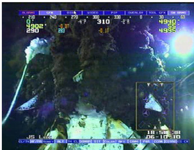
Figure F-1: ROV image of the application of dispersants to oil released above the cut riser pipe using the wand applicator, June 10, 2010 (left side of image). The dispersant plume (white billows) from the wand prior to its entry into the oil release is clearly evident. The dispersant plume path is strongly influenced by the entrained flow near the oil jet, bending almost 70 to 80 degrees from the wand injection direction.
