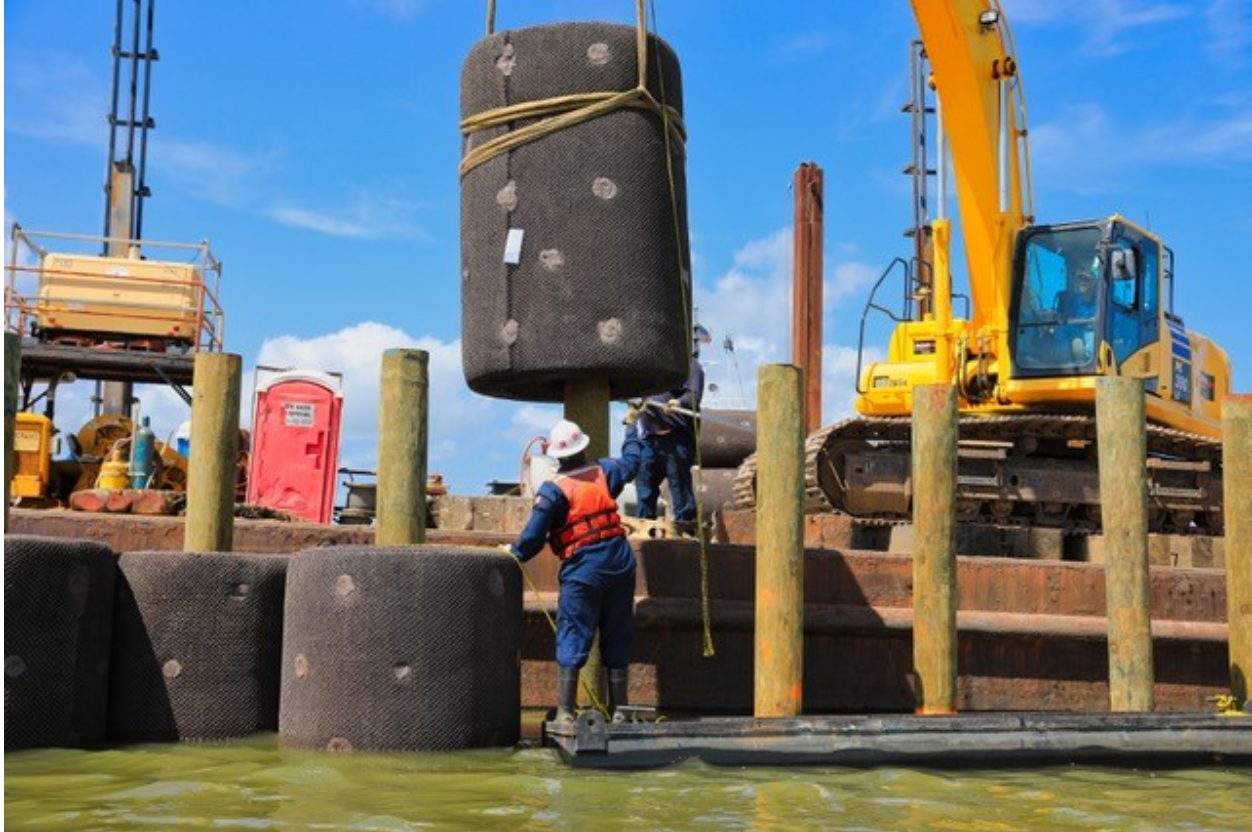
Figure 2. EcoBale unit being placed on a timber pile.
