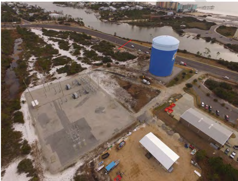
Figure 2. CAST Triage Project Area, looking southeast and showing the approximate location of the proposed water line (in red).
