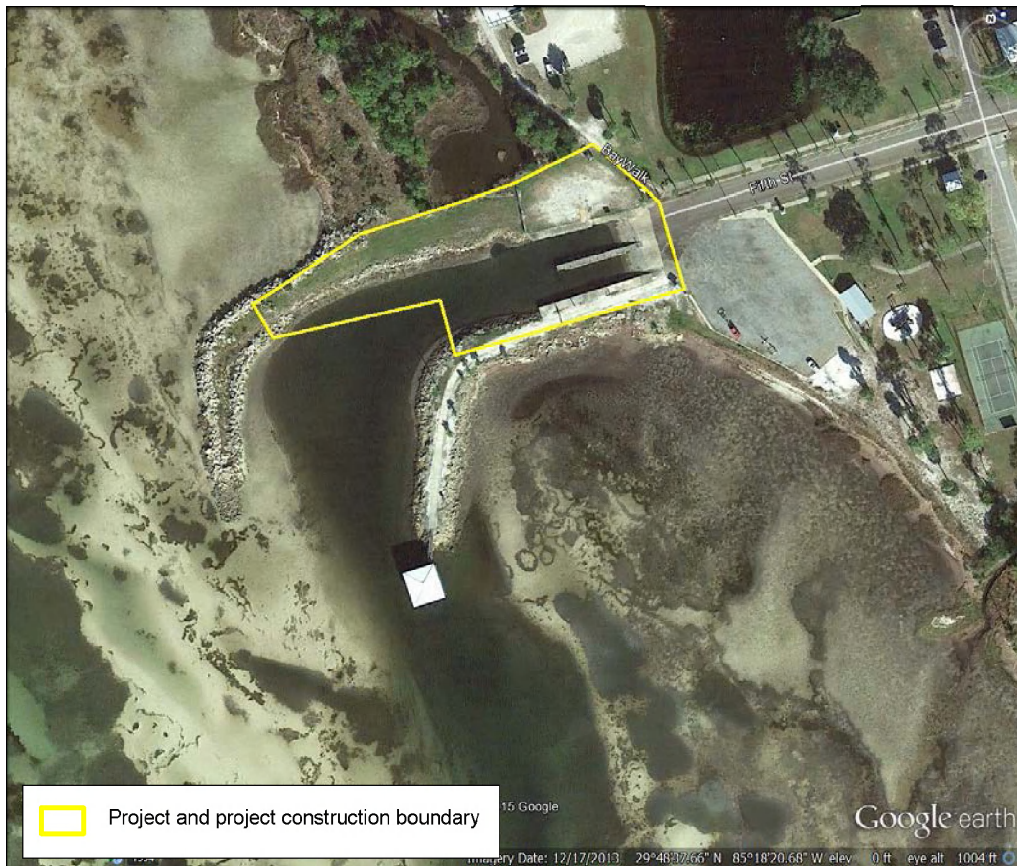
Figure A-3. Location of the Frank Pate Boat Ramp Improvements Project with Described Modification
