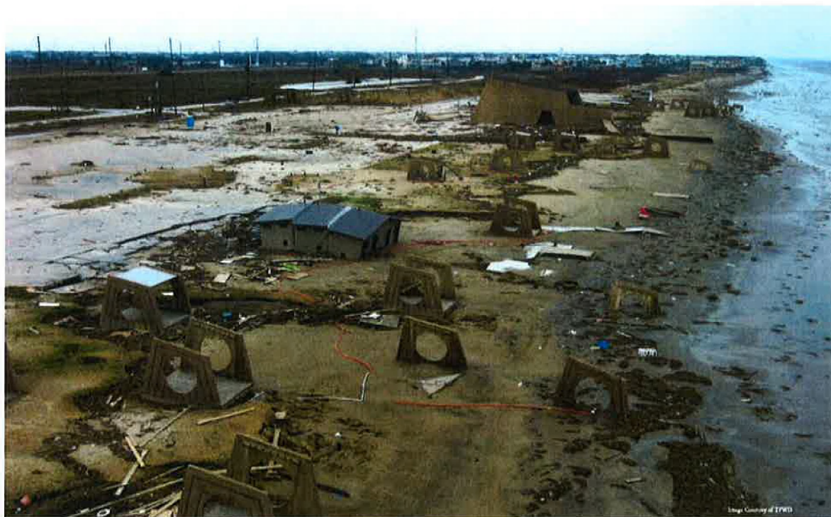
Figure 2. Destruction caused by Hurricane Ike at Galveston Island State Park.
