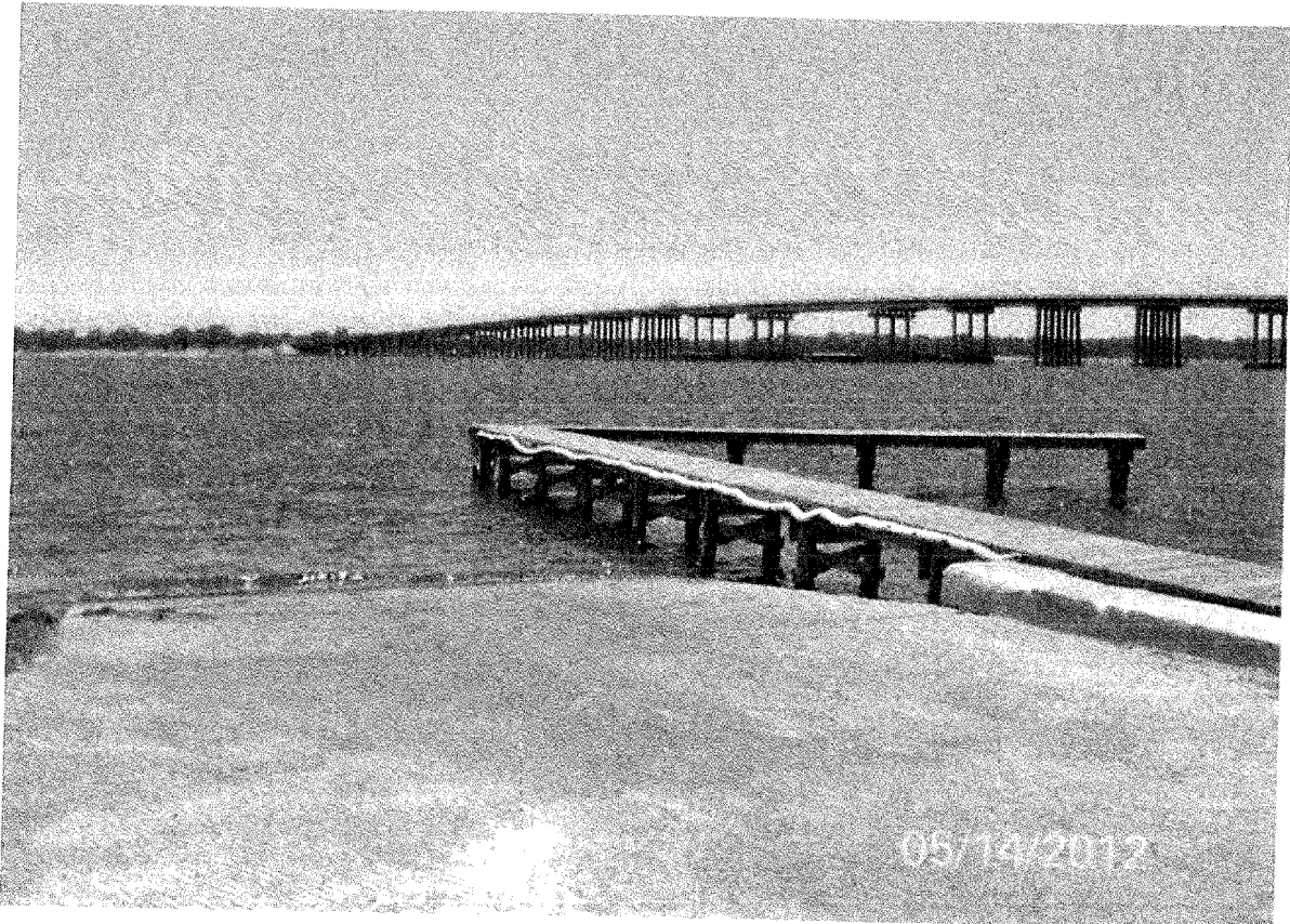
Figure 7. Photo of the proposed project area including the boat ramp and dock that will be repaired as part of the Earl Gilbert action.
