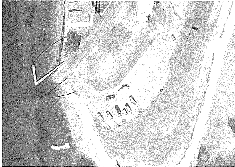
Figure 9. Image of the Earl Gilbert boat ramp with the cofferdam (red open rectangle) and the turbidity curtain (red arc). (©2014, C. Robertson, FL DEP)
