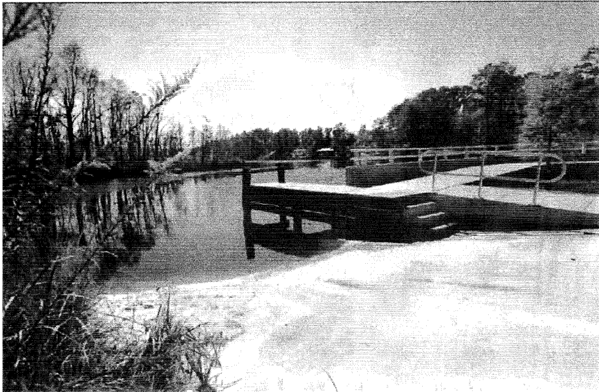
Figure B. A photo of the existing boat ramp and dock.
