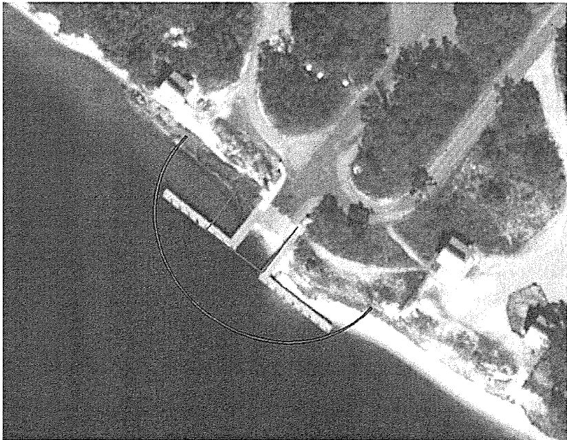
Figure 2. Image of the Big Lagoon State Park boat ramp improvement site with the cofferdam (red open rectangle) and the turbidity curtain (larger red arc). (©2014, C. Robertson, Florida Department of Environmental Protection [FL DEP])
