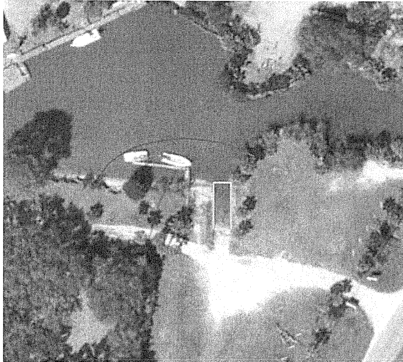
Figure 5. Image of the Indian Creek Park boat ramp improvement site with the cofferdam (green rectangle) and the turbidity curtain (red arc). (©2014, C. Robertson, FL DEP)
