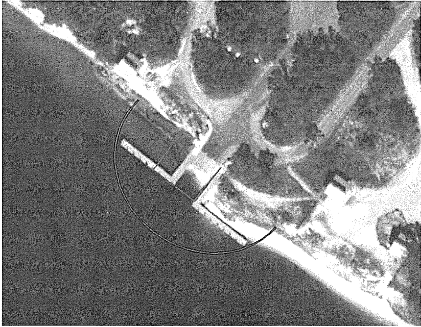
Figure 2. Image of the Big Lagoon State Park boat ramp improvement site with the cofferdam (red open rectangle) and the turbidity curtain (larger red arc). (©2014, C. Robertson, Florida Department of Environmental Protection [FL DEP])
