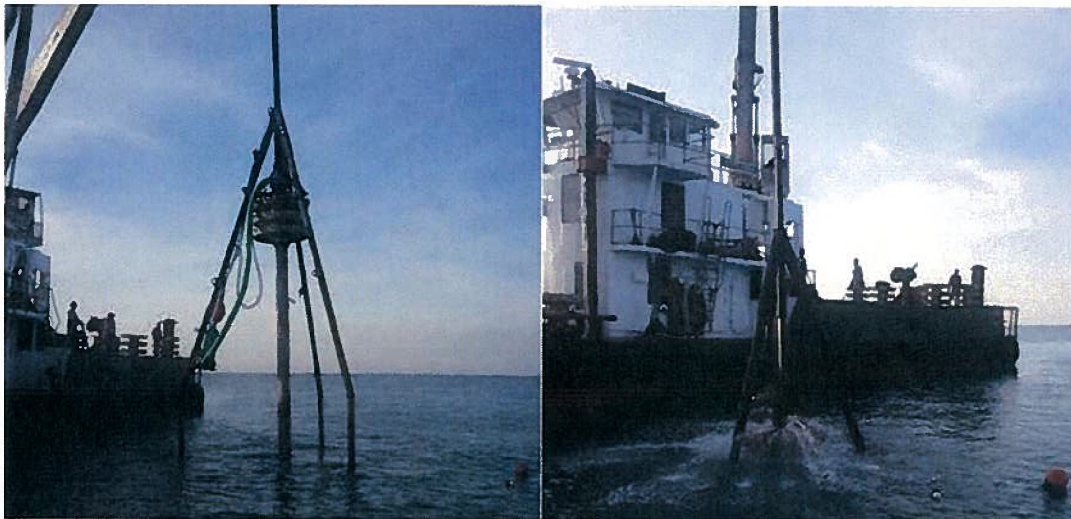
Figure 4. Disk-type reef module deployment with tripod followed by ambient seawater pumping (©2011, Robert Turpin, Escambia County Marine Resources Division)
