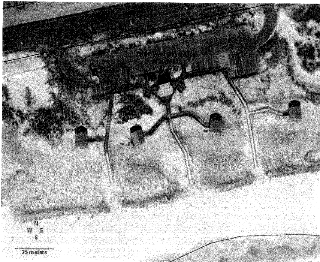
Figure C. Parking lot adjacent to Perdido Key State Park Beach Boardwalk Improvements - western project site.
