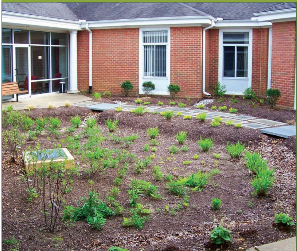
Kramer Center, Centreville, MD Photo courtesy of: McCrone, Inc., Civil Engineers and Surveyors
