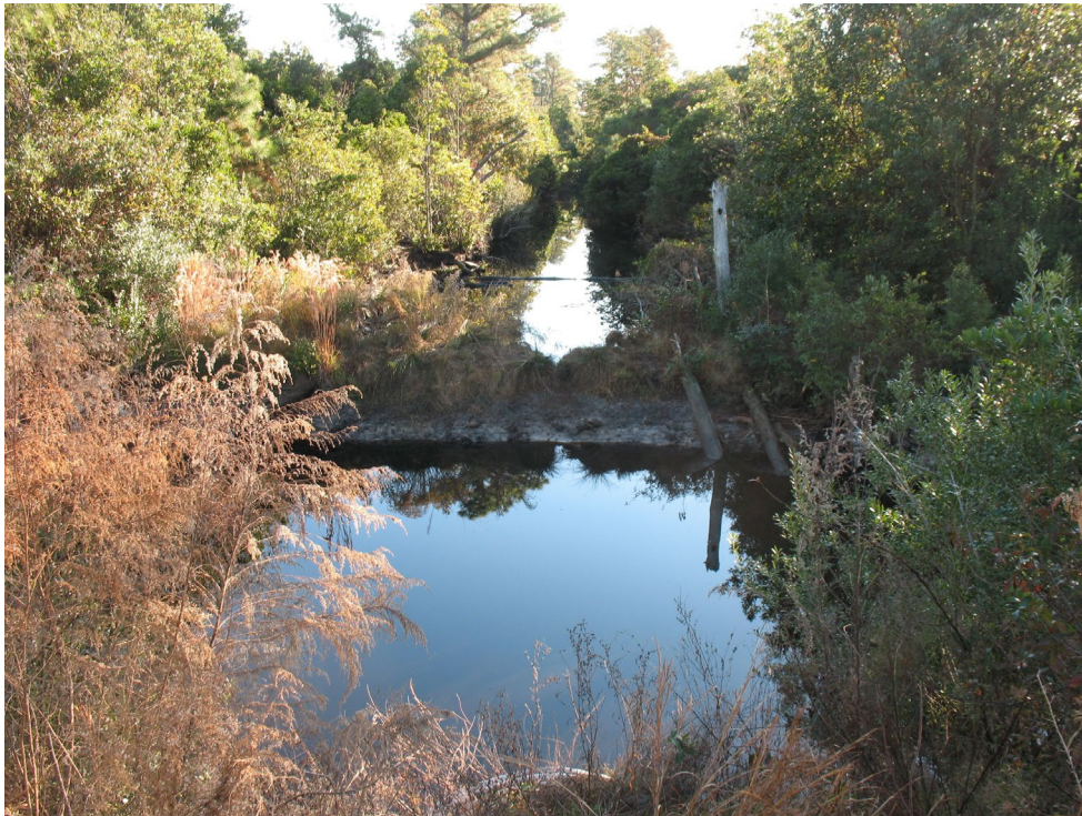
Figure A-29. Earthen plug, built with hand tools, on the far side of J Canal.
