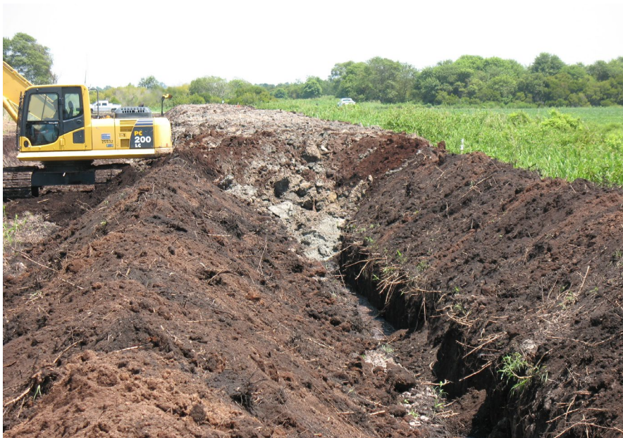
Figure A-26. Clayton Blocks Project cored dike during construction.
