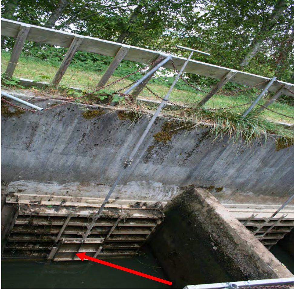
New Tenasillahe Island Tidegate with fish door closed. Photo: USFWS
