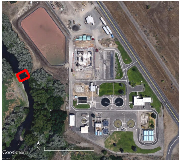
Figure 5. Interrogation site adjacent to the Hermiston Recycled Water Facility (UMW). The red rectangle indicates the location of the PIT array. The river flow is from the bottom to the top of the picture.
