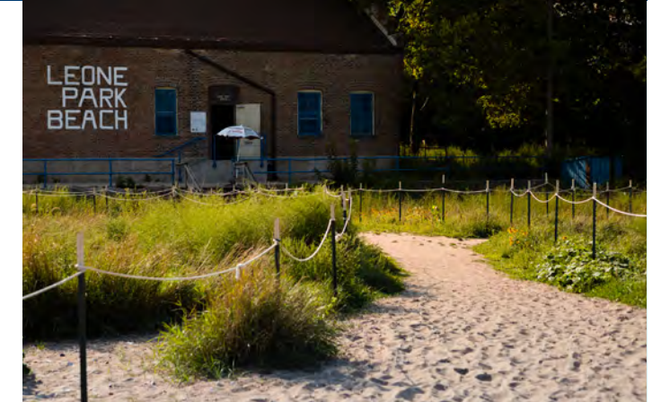
Field house at Leone Park Beach in Chicago.
