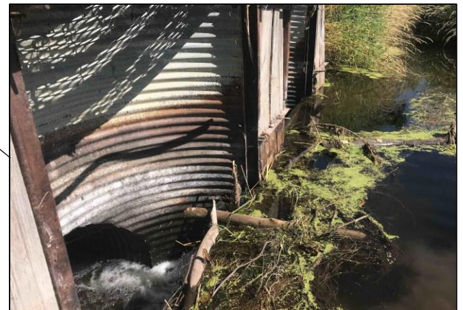
Relic check dam, altering natural flow and sediment regimes and preventing fish migration.
