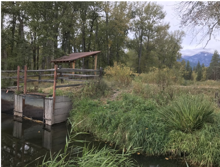
Figure 3-6. The water control structure (foreground) and Viewing structure (background) along the paved trail in the Refuge WVA.
