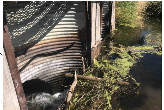
Relic check dam, altering natural flow and sediment regimes and preventing fish migration.
